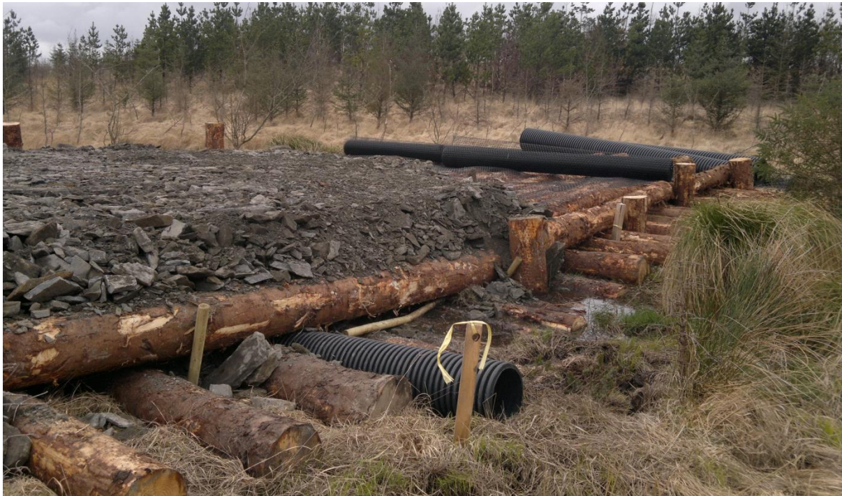
Figure 3-8 Lightweight floated road in place across flush area
