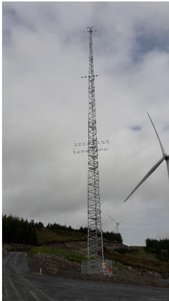
Figure 3-32 Typical Permanent Meteorological Mast on a Wind Farm
