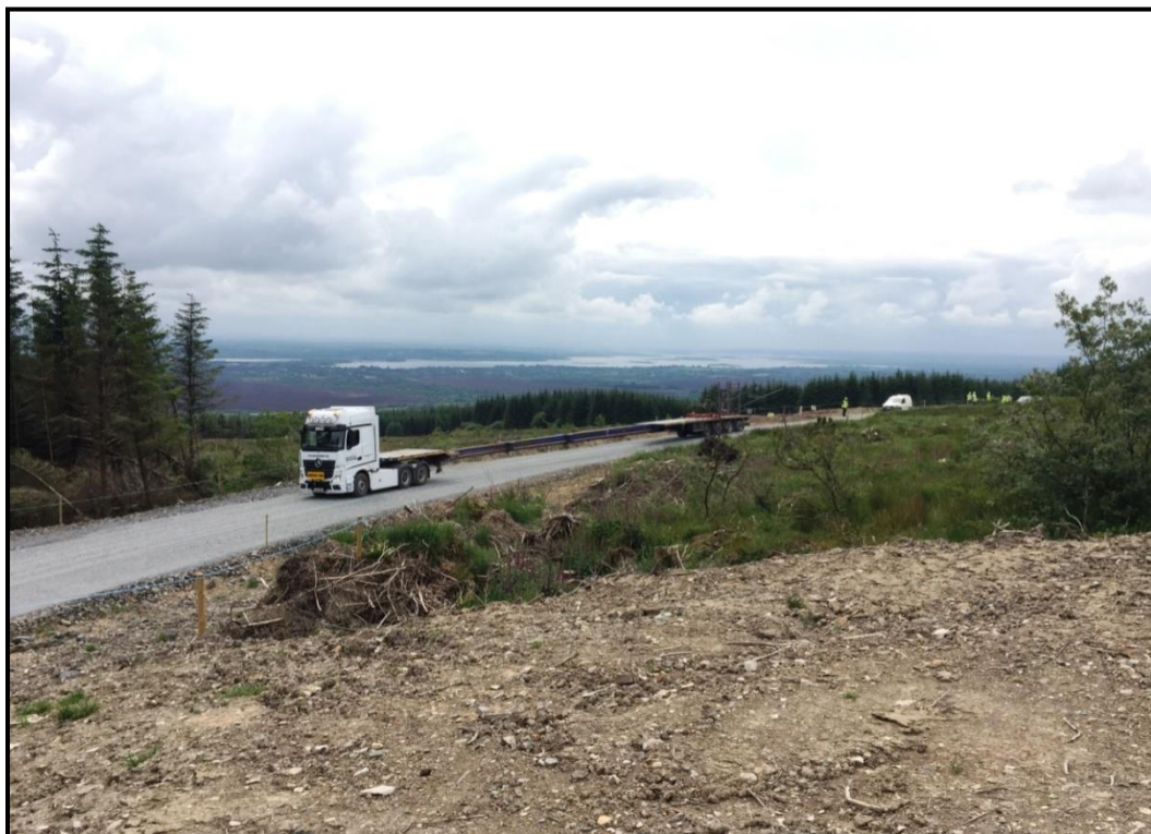
Figure 3-3 Typical upgraded forestry road on a wind farm
