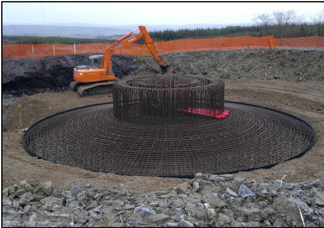
Figure 3-20 Typical construction of a wind turbine base
