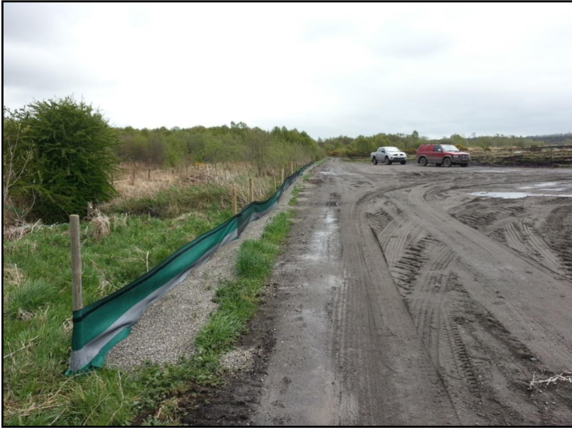
Figure 3-11 Silt curtain containment along existing roads near existing drains or watercourses
