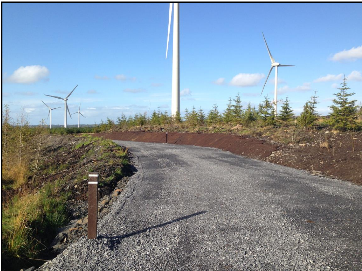
Figure 3-5 Typical new excavated road on a wind farm
