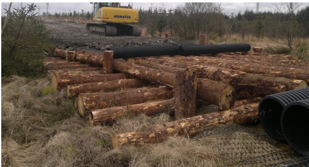
Figure 3-7 Typical Log Road in process of construction on a Wind Farm
