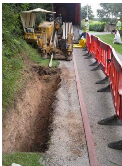
Figure 3-31 Typical directional drilling rig and launch pit
