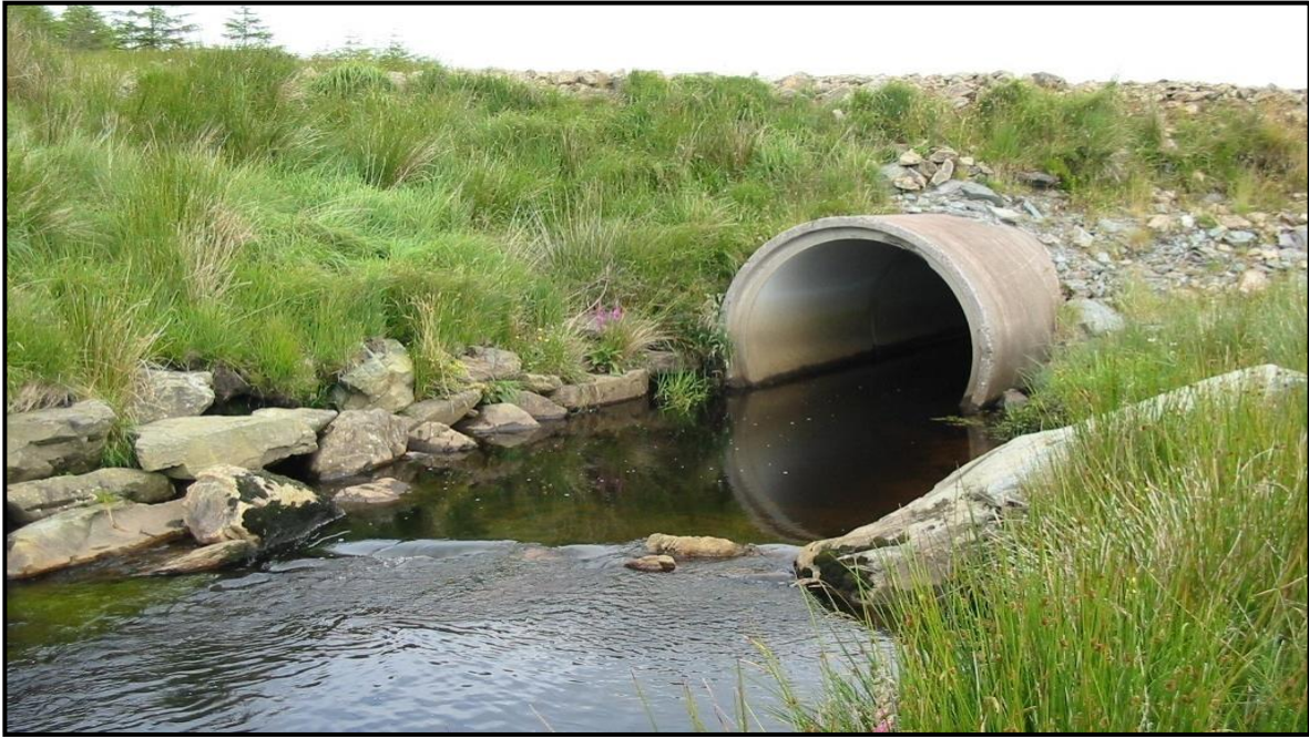
Figure 3-9 Typical drainage channel crossing
