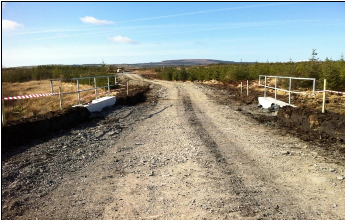
Figure 3-10 Dirty water containment at existing drains or watercourse crossings
