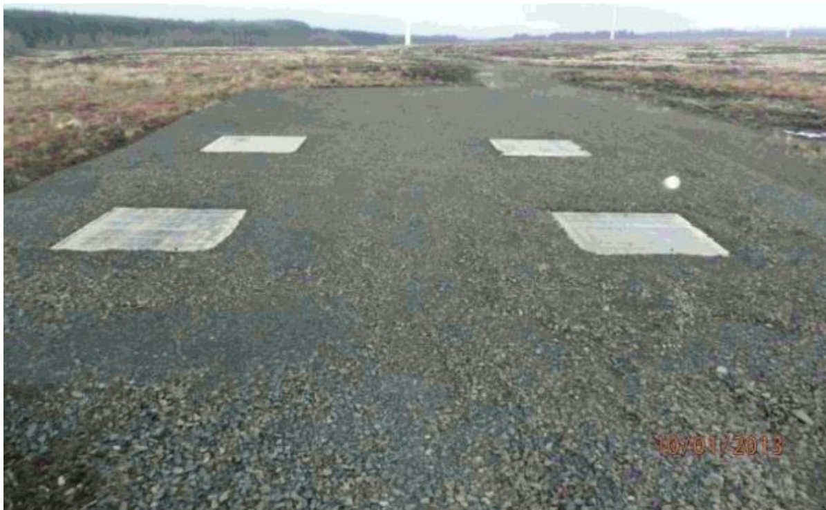
Figure 3-19 Typical Floating/Piled Hardstand Option
