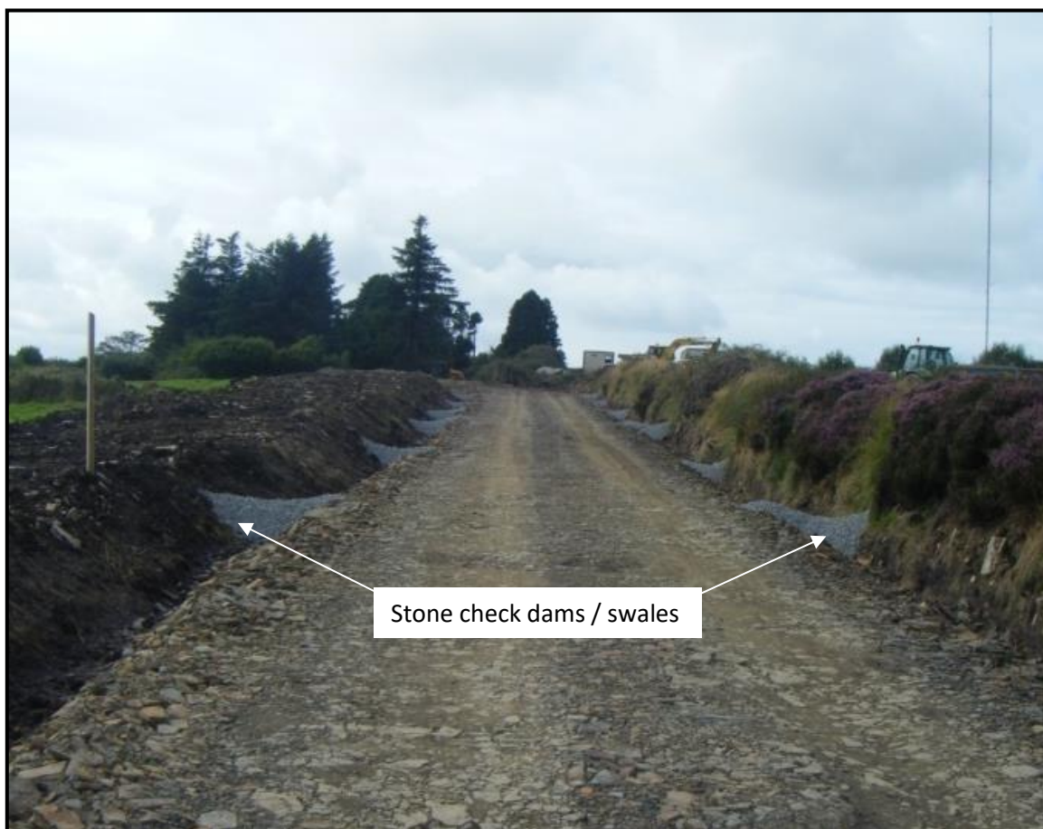
Figure 3-37 Examples of check dams along roadside drainage channels
