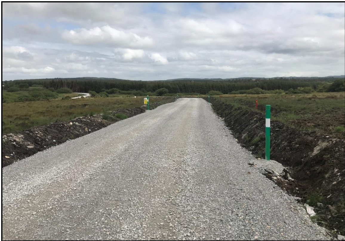
Figure 3-6 Typical floated road on a wind farm
