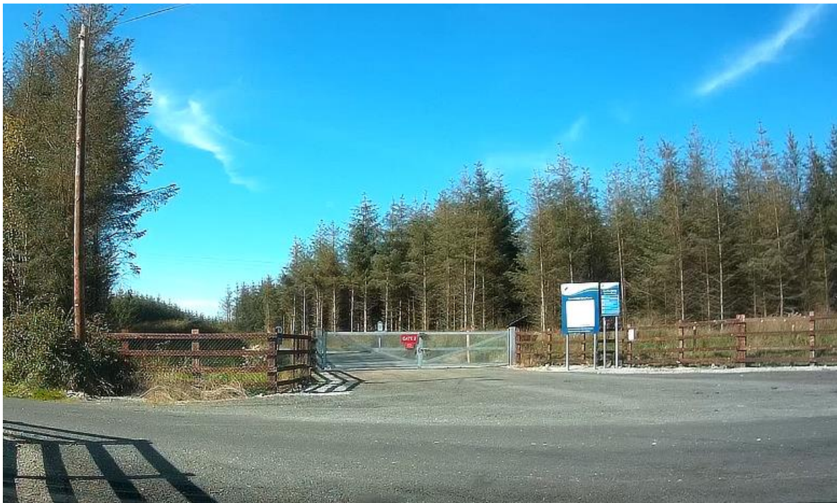
Figure 3-1 Typical Wind Farm Entrance
