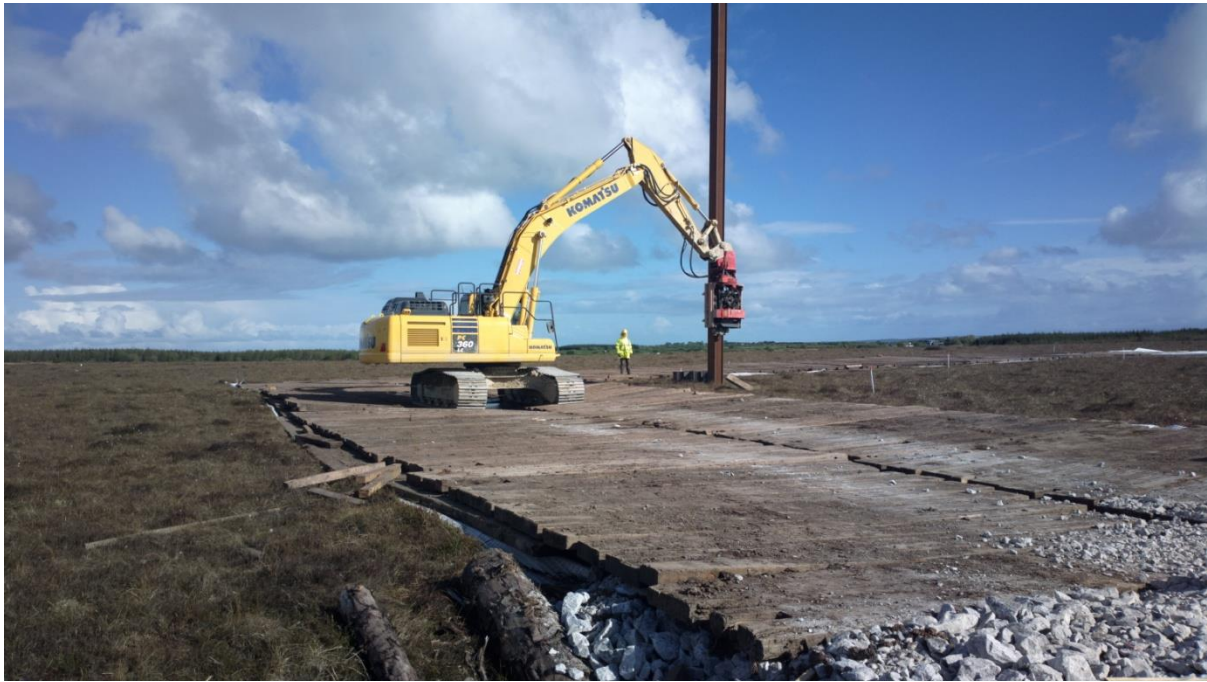
Figure 3-16 Sheet Pile Installation
