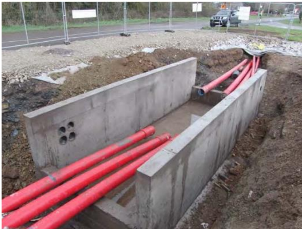
Figure 3-26 Typical joint bay construction
