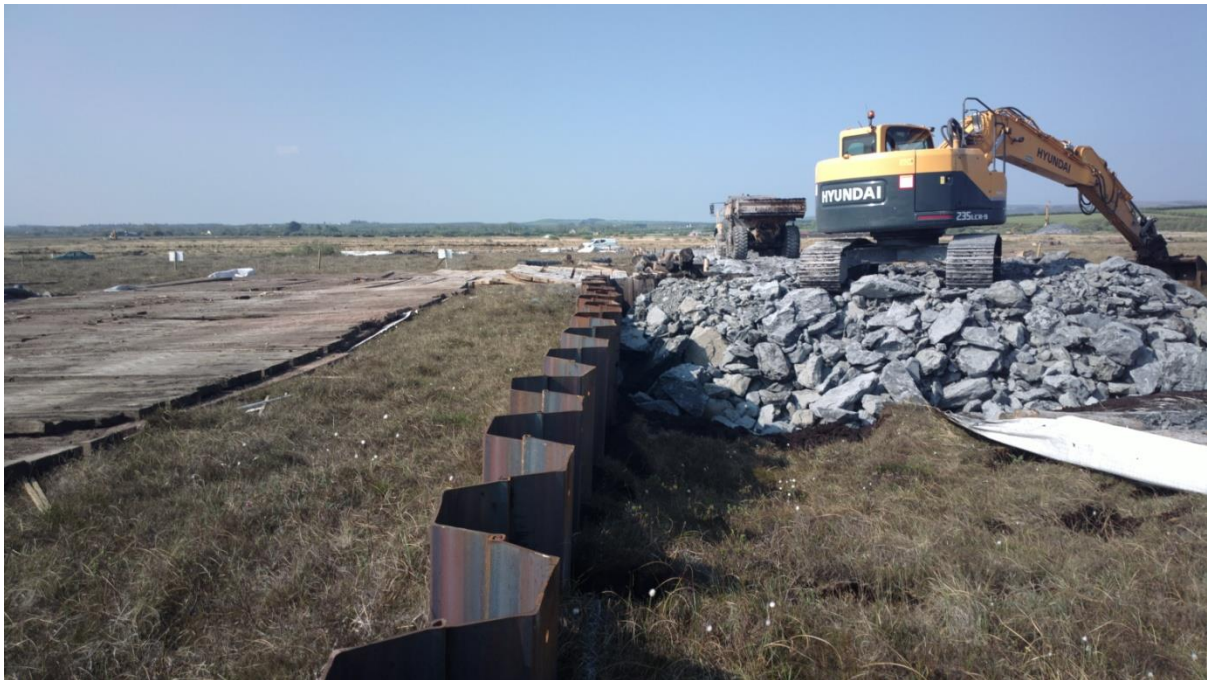
Figure 3-17 Excavating beside the Sheet Pile Cofferdam
